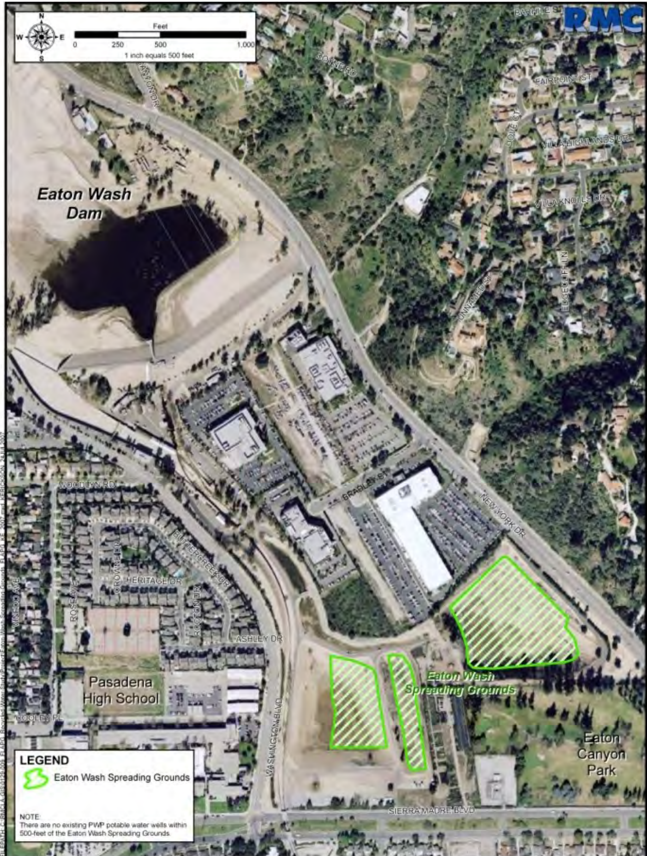
Figure 14: Eaton Wash Spreading Grounds and Wells
