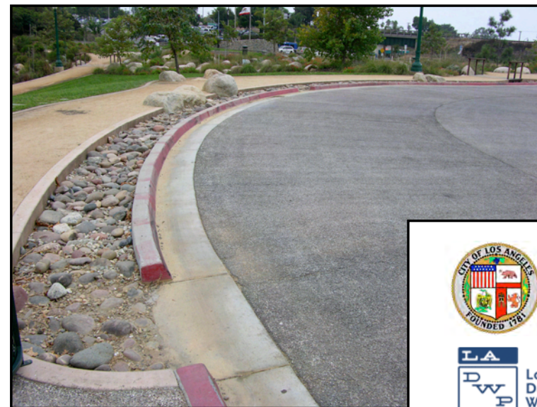
SWALE AT PAVING
