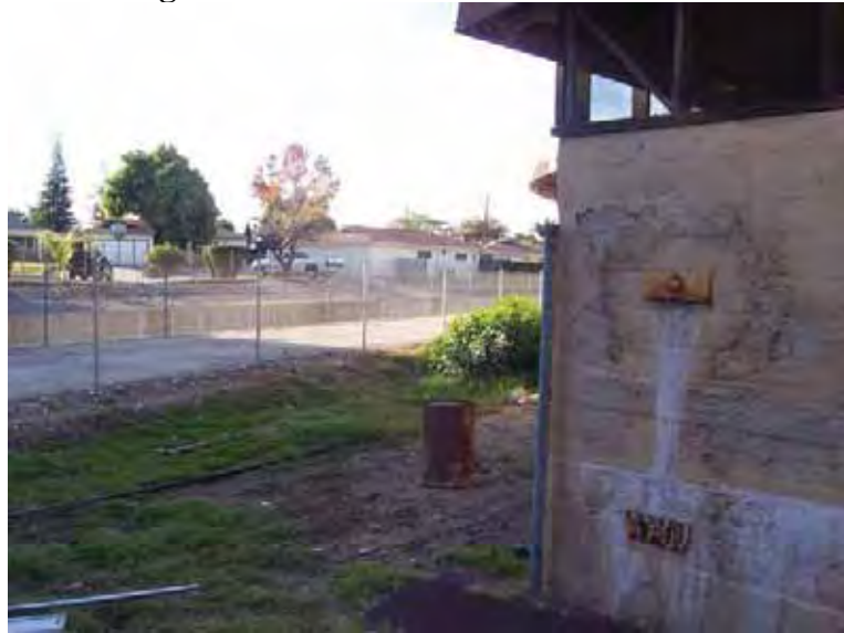
Figure 4-22: Site 10 Little Dalton Wash
